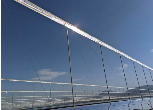
Source: Puerto Errado 2 liner Fresnel mirror power plant, Spain
