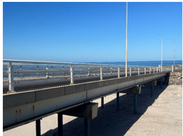
Figure 10: West Beach Bridge
